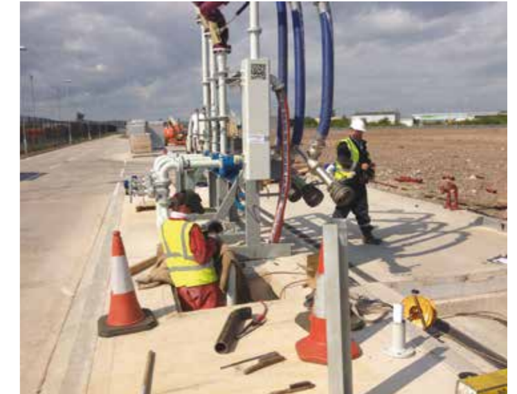
Installation of 3 arm bottom loading skid
