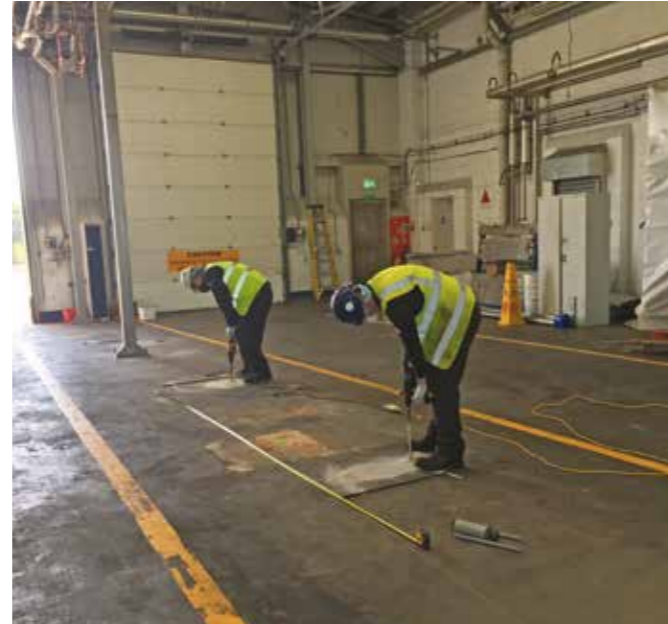
Drilling Floor ready for platform column install
