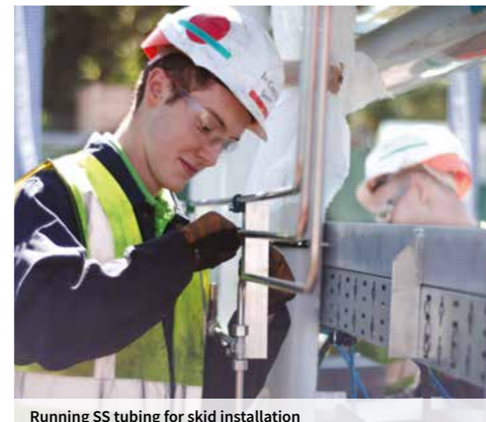
Running SS tubing for skid installation
