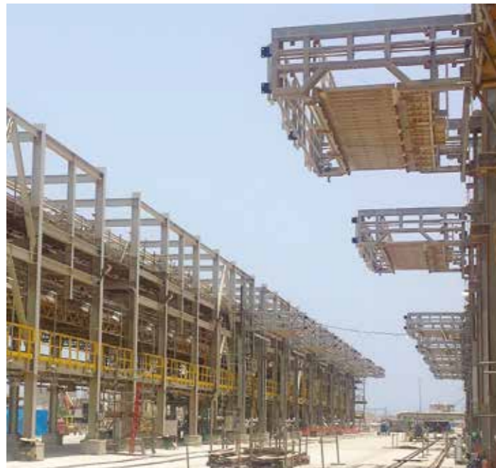
30 x 6m Custom Velp designed for both road and rail tank cars - Saudi Arabia - Chemical Industry
