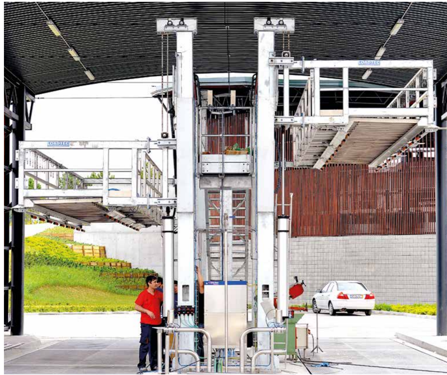
2 x 10m Pneumatic VELP showing full height range - Portugal - Wine Industry
