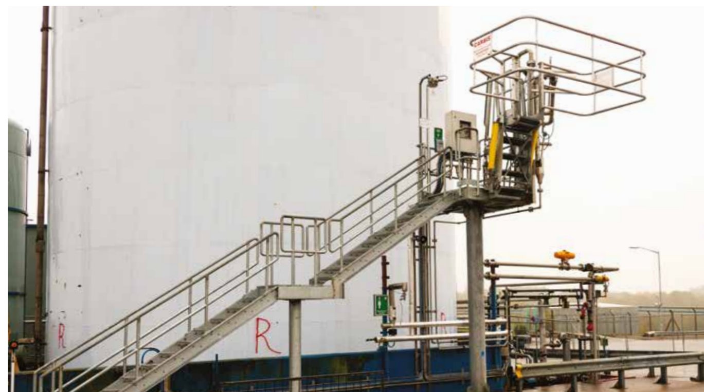
Fixed Access Platform with 5 step folding stair and top loading arm - UK - Chemical Industry
