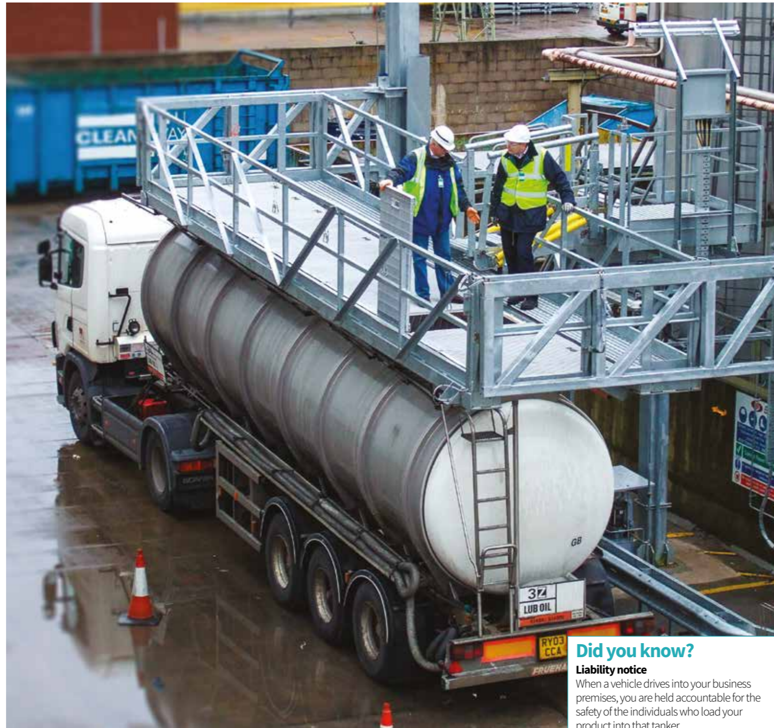
10m Hydraulically Actuated VELP with wide flip up panels - Wales
