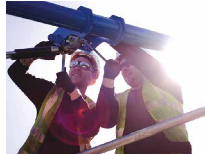
Balance adjustment for loading arm
