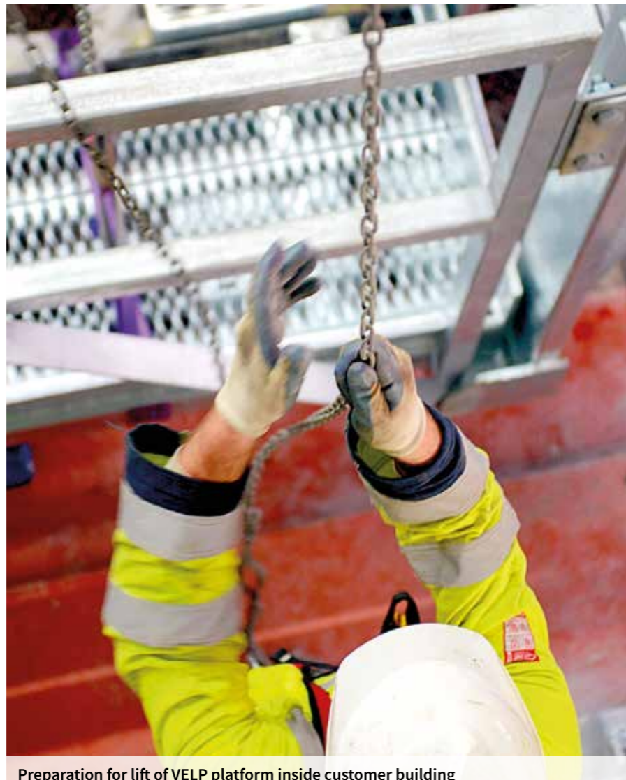
Preparation for lift of VLP platform inside customer building
