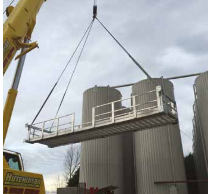
Installation of VLP Cage section
