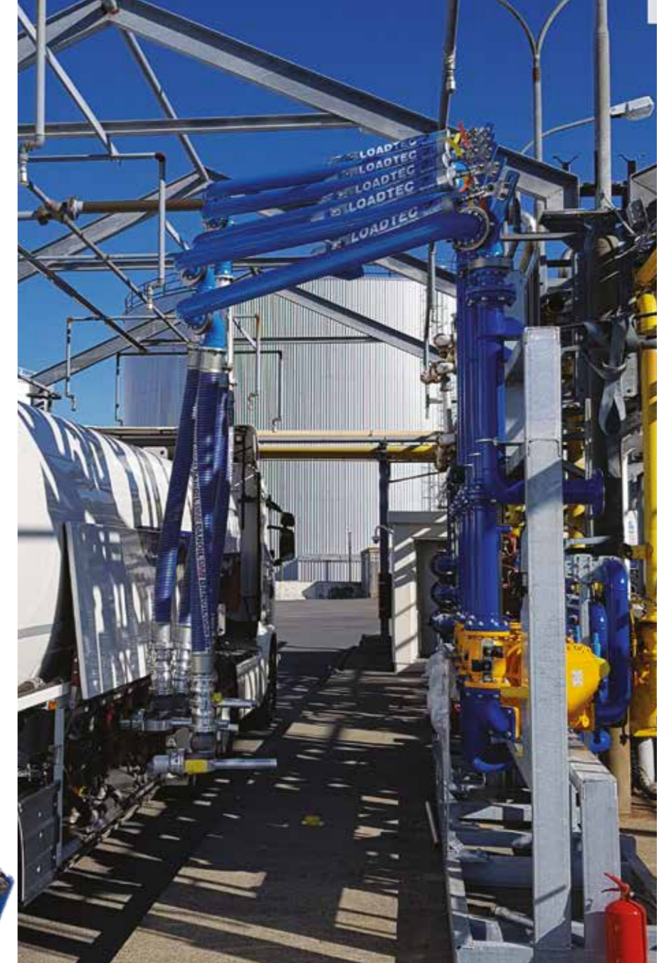
Multiple bottom hose loading arms with crossover for fuels loading - Iceland - Fuels Industry
