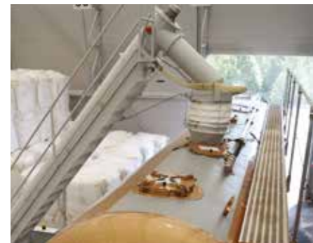
Filling with a capacity of 80 m 3 per hour
