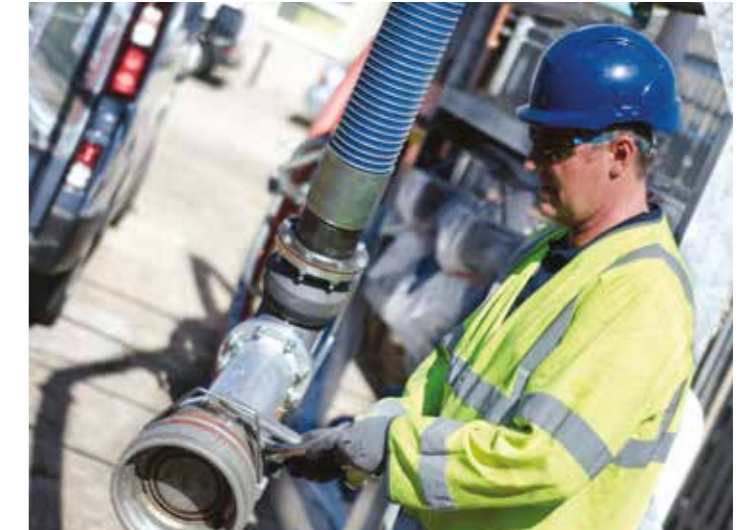
Function check for bottom hose loading arm
