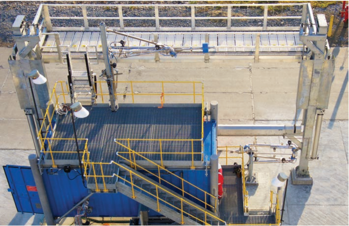
10m VELD pneumatically powered, with top loading and bottom unloading arms, with duty and standby metering skid built into weather proof container subject to extreme sub-zero temperatures. Loading and unloading Artic Diesel in remote locations. Russia- Fuel industry
