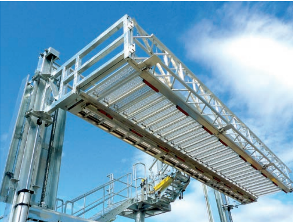
VELP from below showing the rubber bumpers of the tanker detection flaps - UK - Chemical Industry
