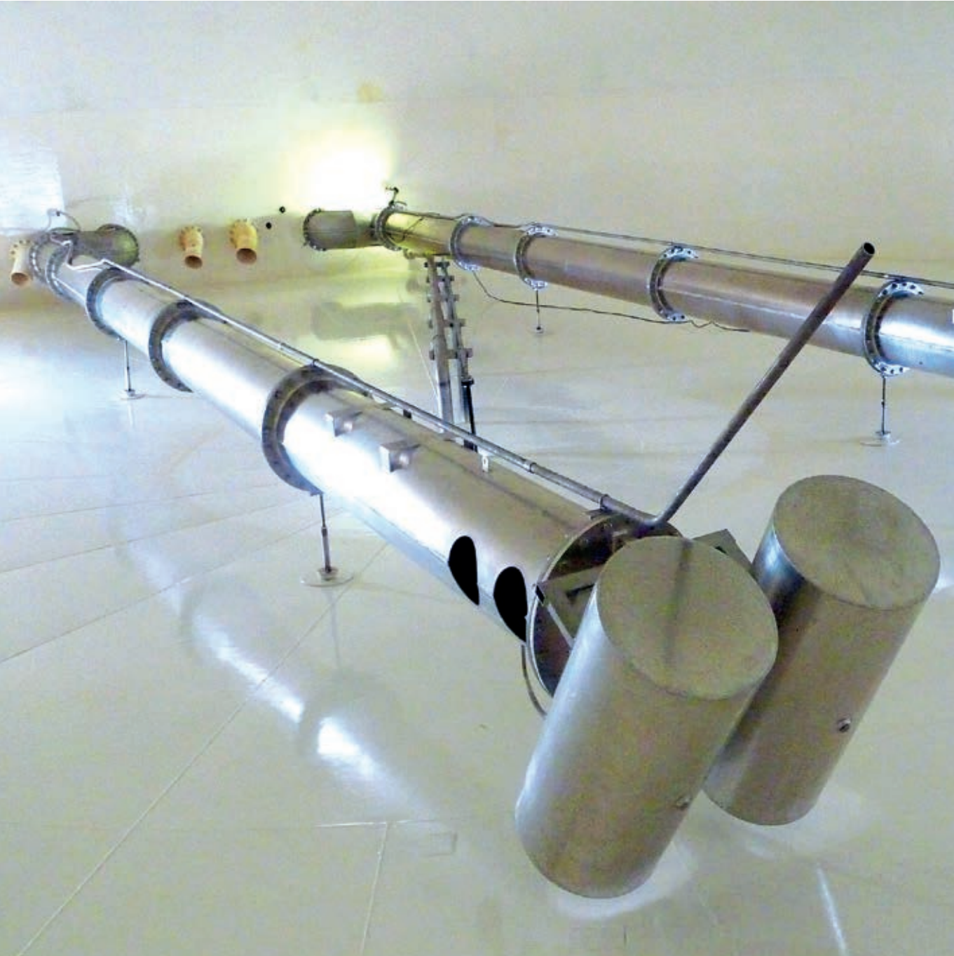
2 x 20" x 15m long Stainless Steel Floating Suctions inside a storage tank ready for Jet Fuel - UK - Aviation
