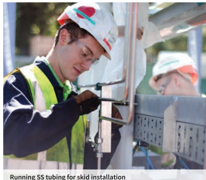
Running SS tubing for skid installation
