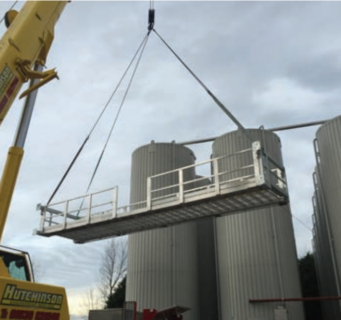
Installation of VEP Cage section
