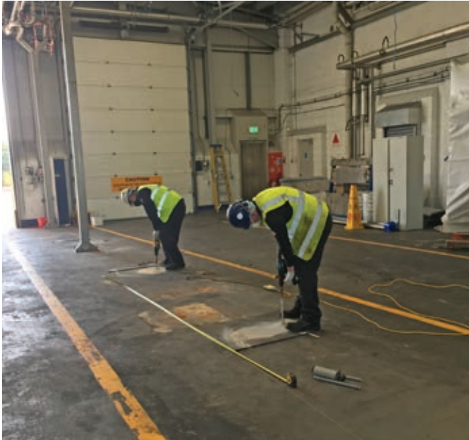
Drilling Floor ready for platform column install
