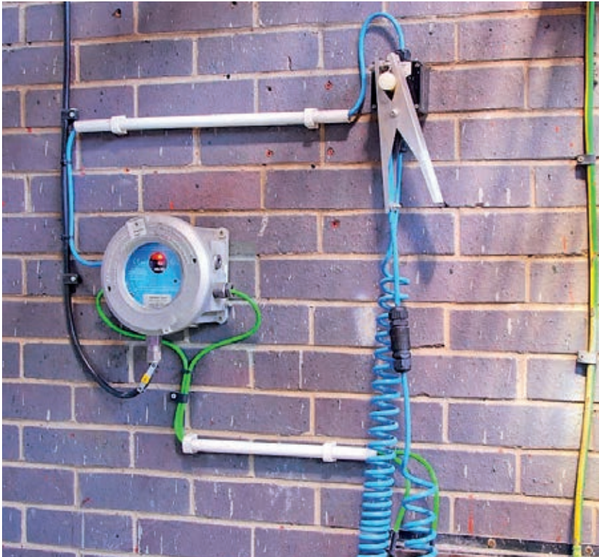
An example set up of tanker earthing with tanker clamp connected to its parking adapter.
