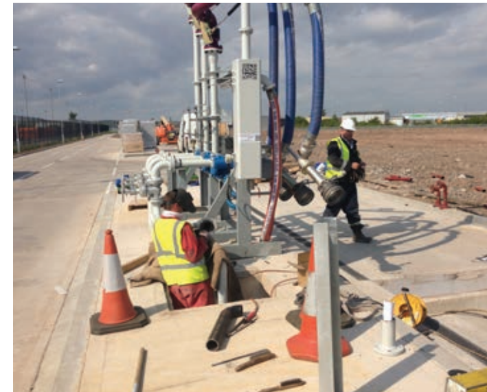
Installation of 3 arm bottom loading skid
