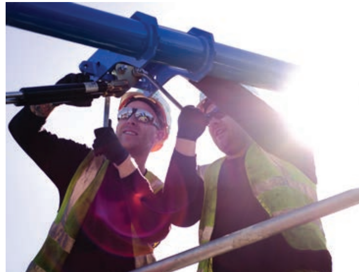
Balance adjustment for loading arm
