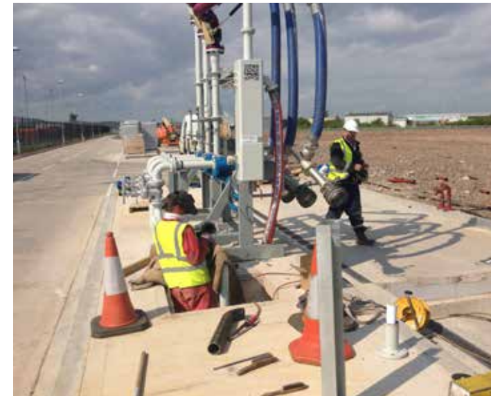
Installation of 3 arm bottom loading skid
