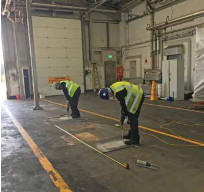
Drilling Floor ready for platform column install
