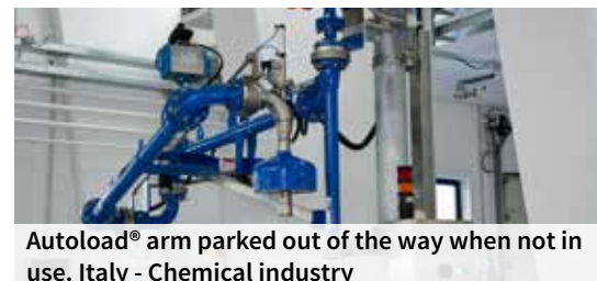
Autoload® PTFE lined IBC loading arm, electrically actuated with control valves and Titanium Drop pipe with anti-drip valve for clean loading. - Italy - Chemical industry
