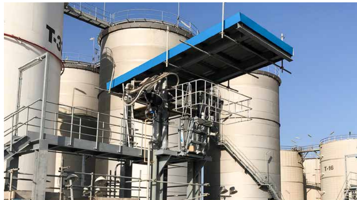
Custom designed fixed access platform with canopy for operator protection, 2 x top loading arm with vapour return and folding stair - Saudi Arabia - Chemical Industry
