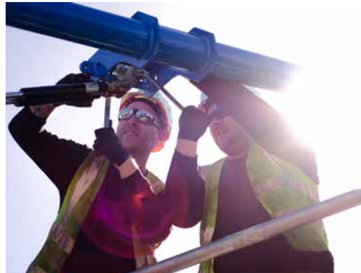
Balance adjustment for loading arm
