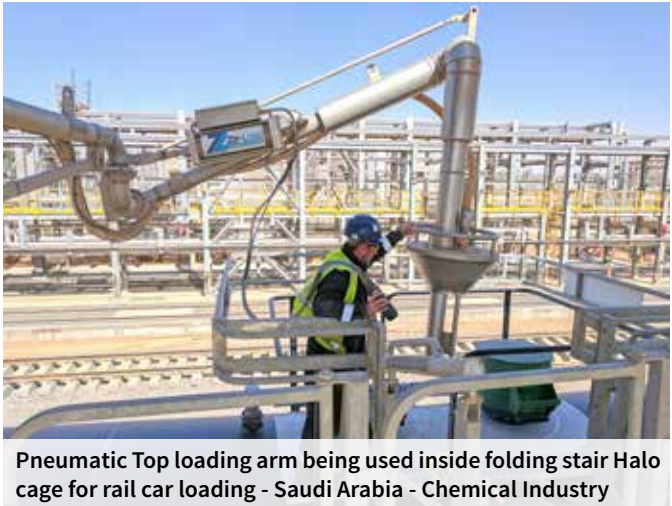
Track mounted Gangways with Loading Arm and meter skids for Acid - Saudi Arabia - Chemical Industry
