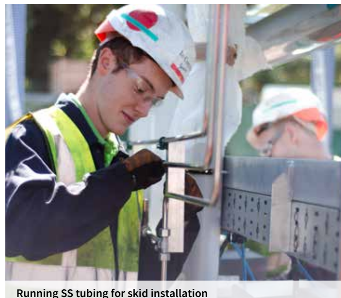
Running SS tubing for skid installation
