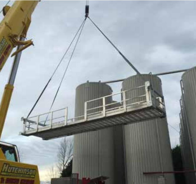
Installation of VELP Cage section
